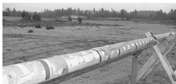
Figure 22. Trial 4 shells wrapped and ready to be pulled into steel pipe.
