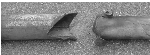
Figure 21. Damage at location of the last shell of those assembled within pipe (Trial 3).
