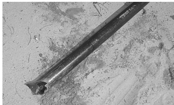
Figure 11. Damage at end of pipe (30-cm length missing).
